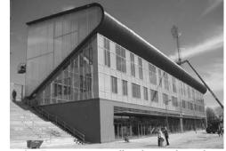
Figure 2: Transparent windbreak on the side of the Fredrikstad Stadium in Norway.
